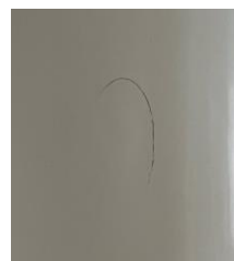
Reappearance of crack around overflow
