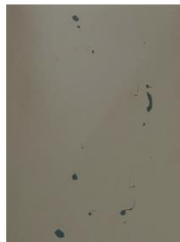
Chips on the tub bottom
