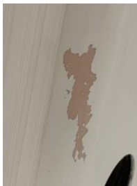
Scratch after installing ceramic walls
