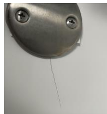
Reappearance of crack around overflow
